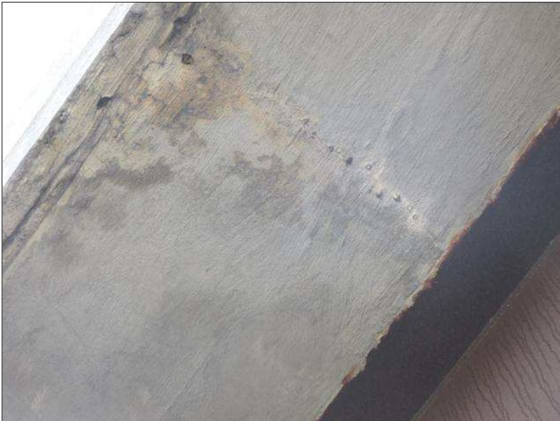
CRACKS IN BOTH OVERHANGS
