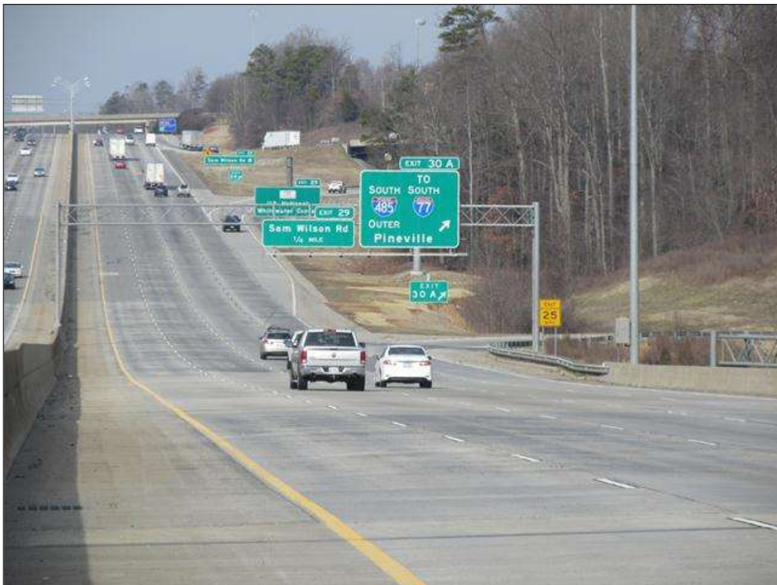
RAMPS LOOKING SOUTH
