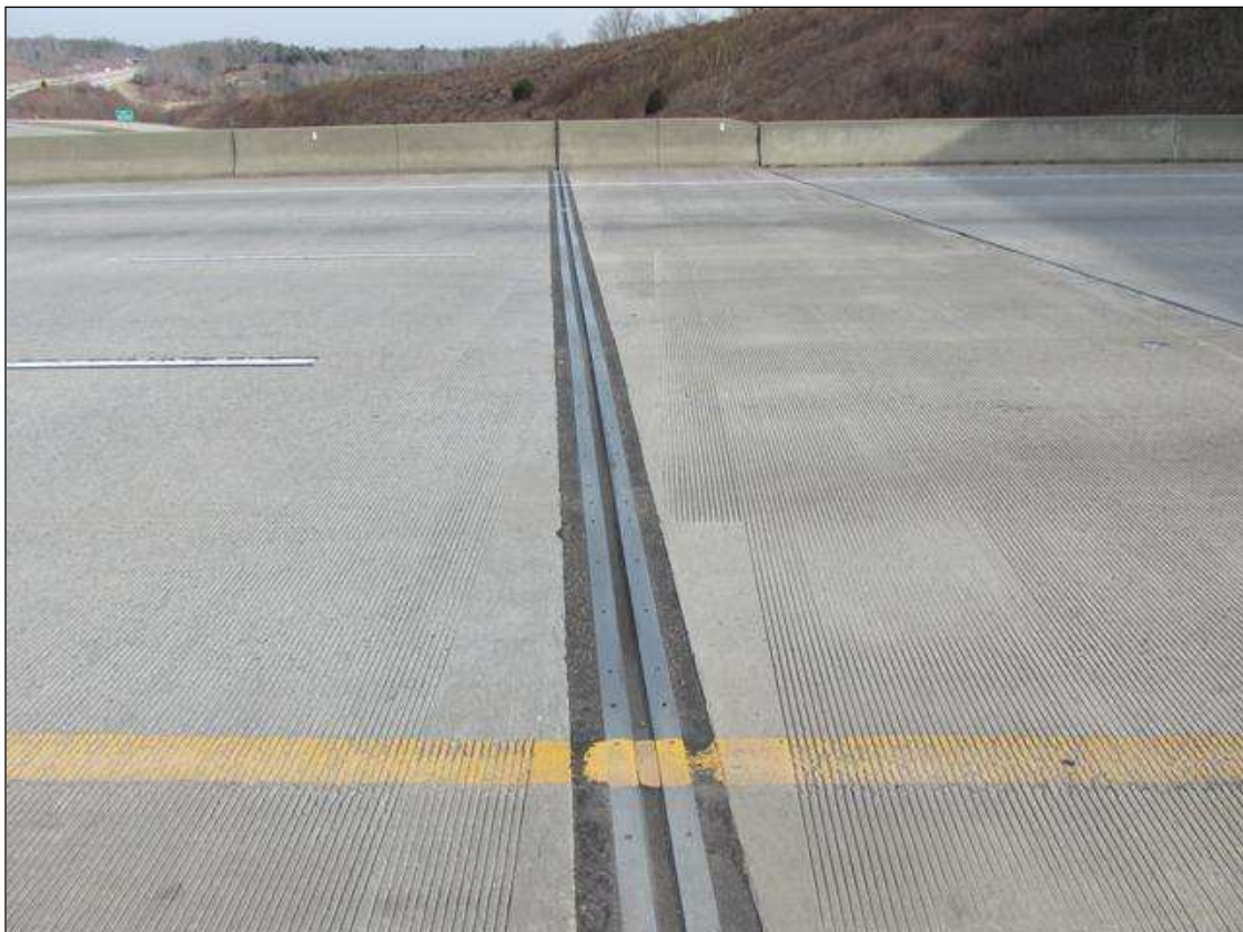
EXP. JOINTS AT BOTH ABUTMENTS
