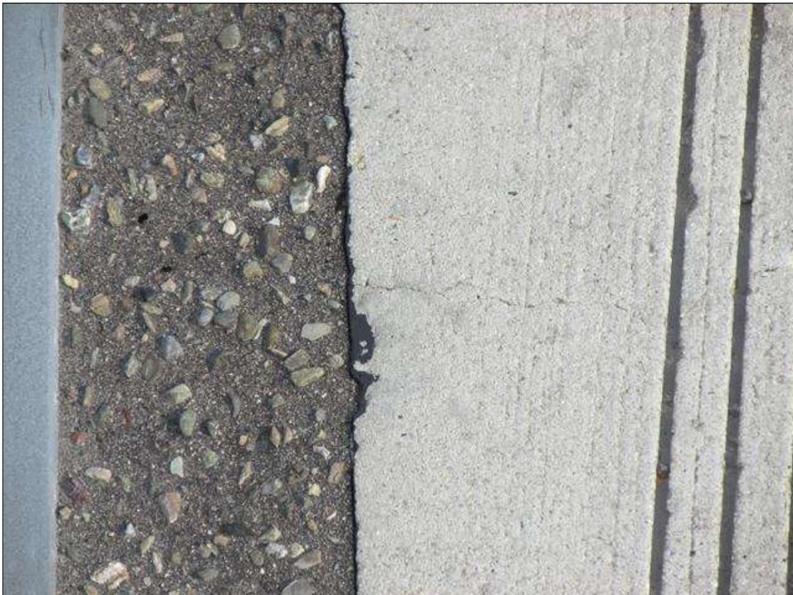
HL CRACKS IN SPAN ENDS
