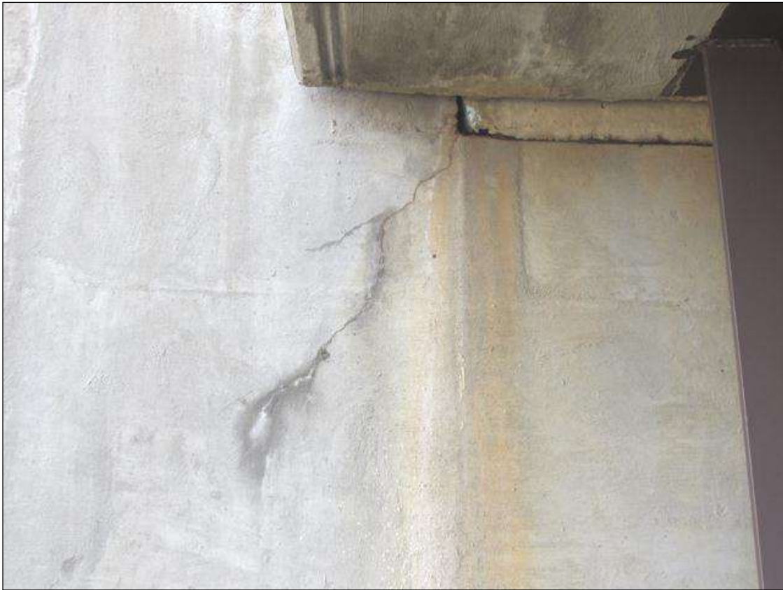
HL DIAGNOL CRACKS IN BOTH ABUTMENT BACKWALLS
