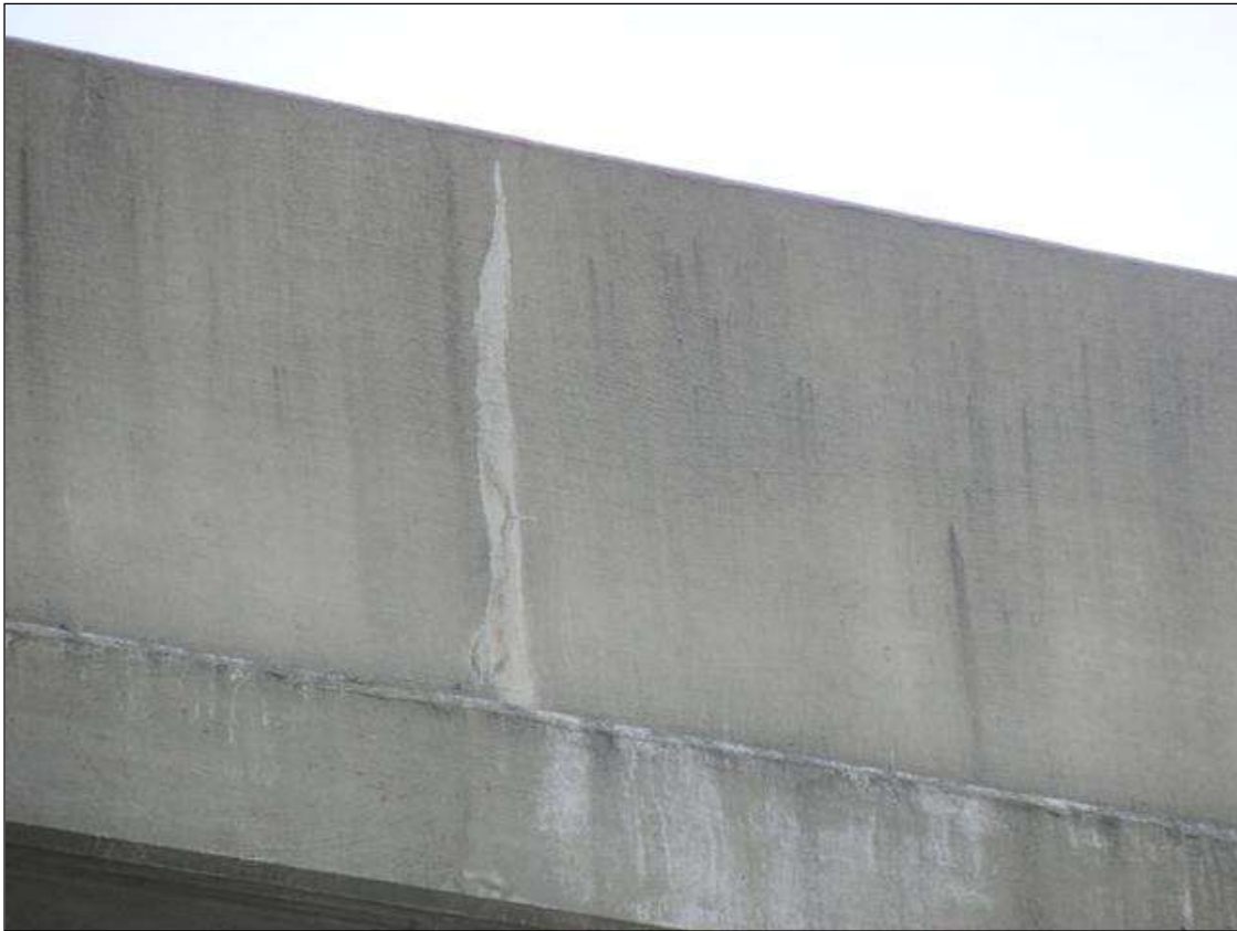
CRACKS IN BOTH RAILS
