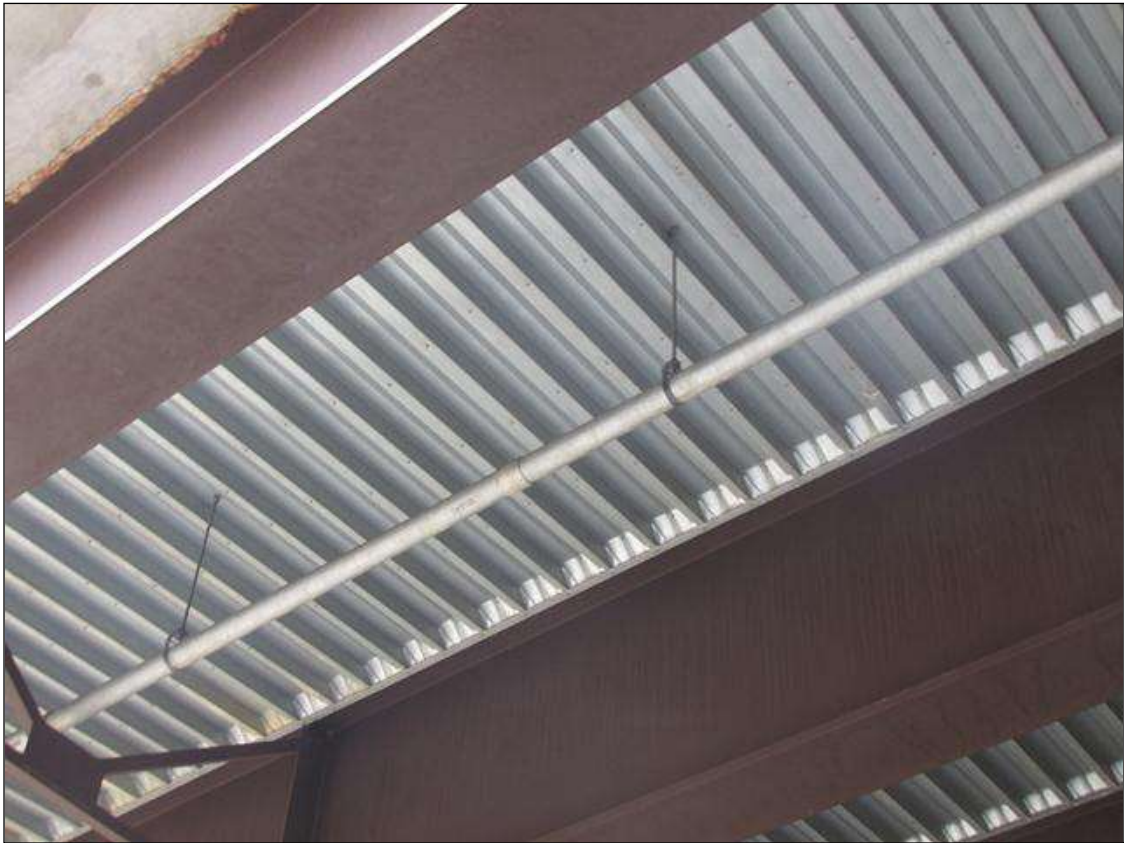
1 - 4" UTILITY IN BAY # 13
